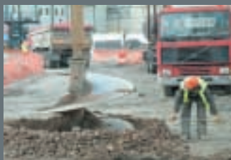
One of the 300 piles.
