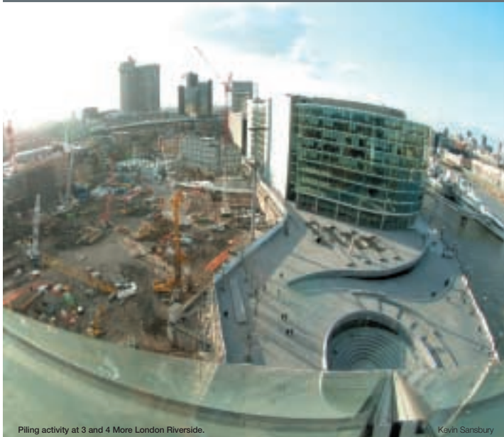
Piling activity at 3 and 4 More London Riverside.
